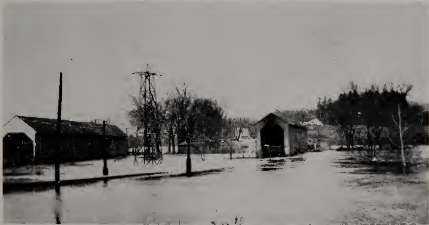
The covered bridge of 1874 and the P.V. Railroad bridge over the Baker River on Route 3, photographed during the flood of 1927.
